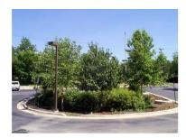
This rain garden is helping to address storm water concerns in a parking lot. It will help collect potential pollutants such as motor oil before the runoff water moves untreated through the storm drain system and into our local creeks, streams, rivers and lakes.
